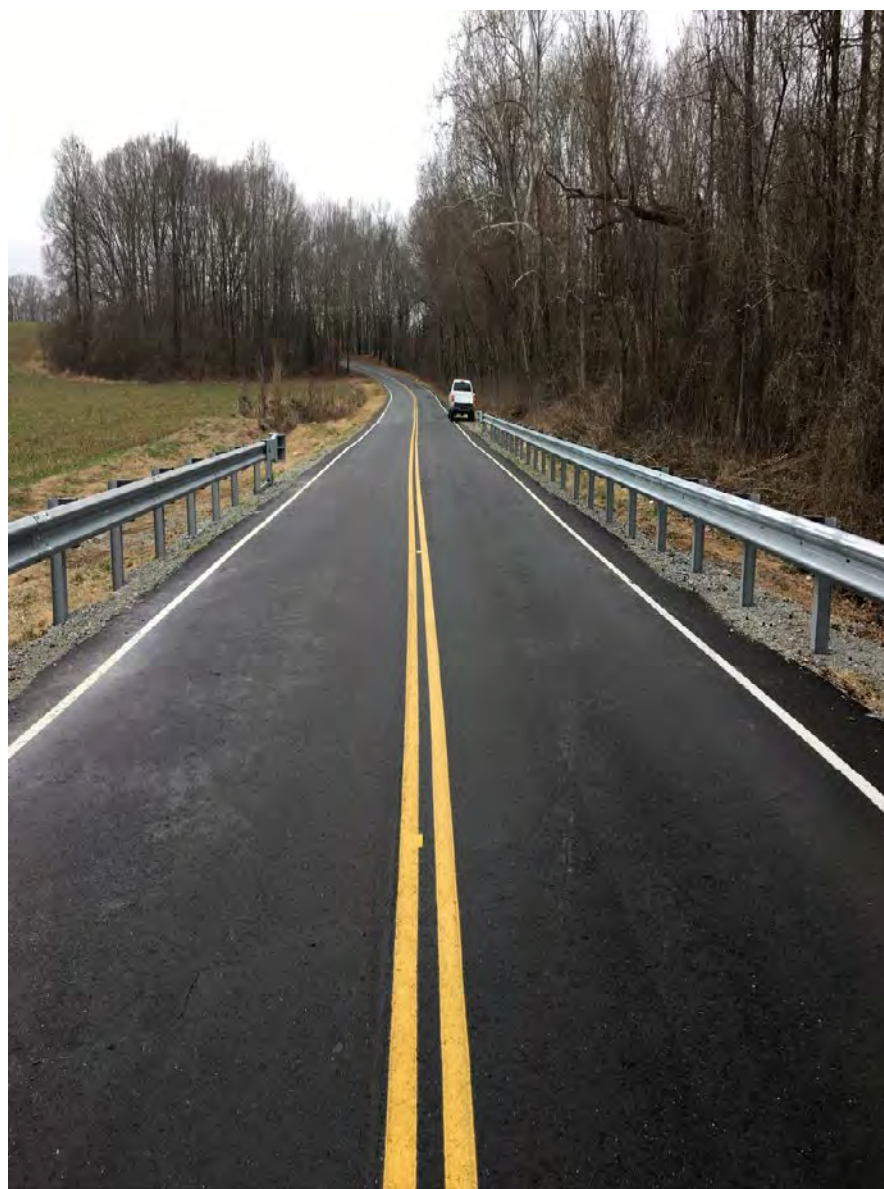
Westbound from Bridge
