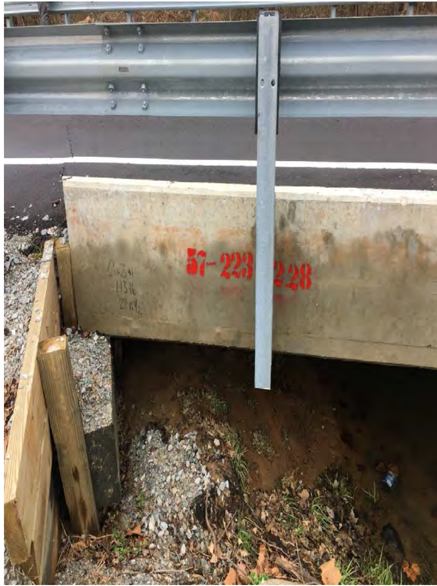
Connection to West Abutment on Inlet Side
