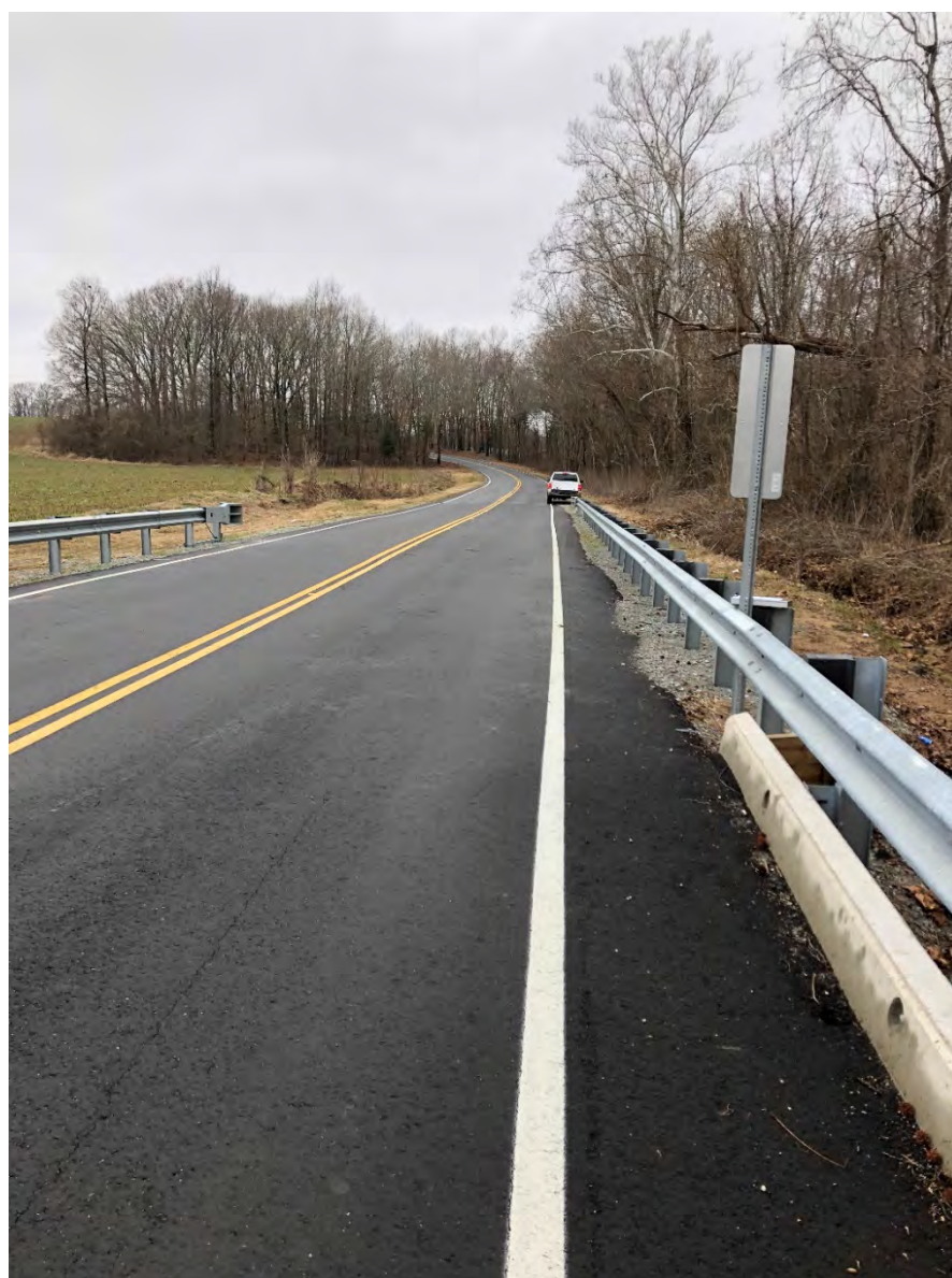
Looking West from Bridge
