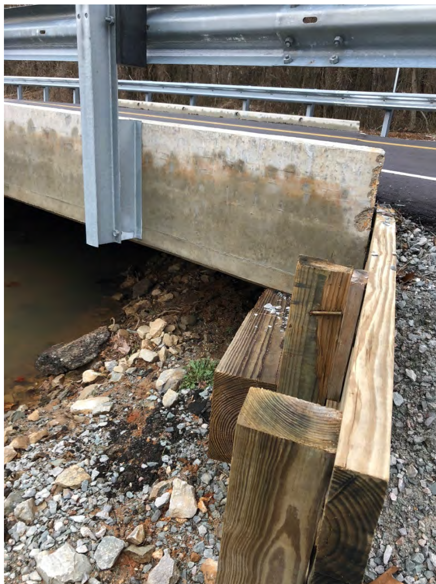
Connection to East Abutment on Inlet Side
