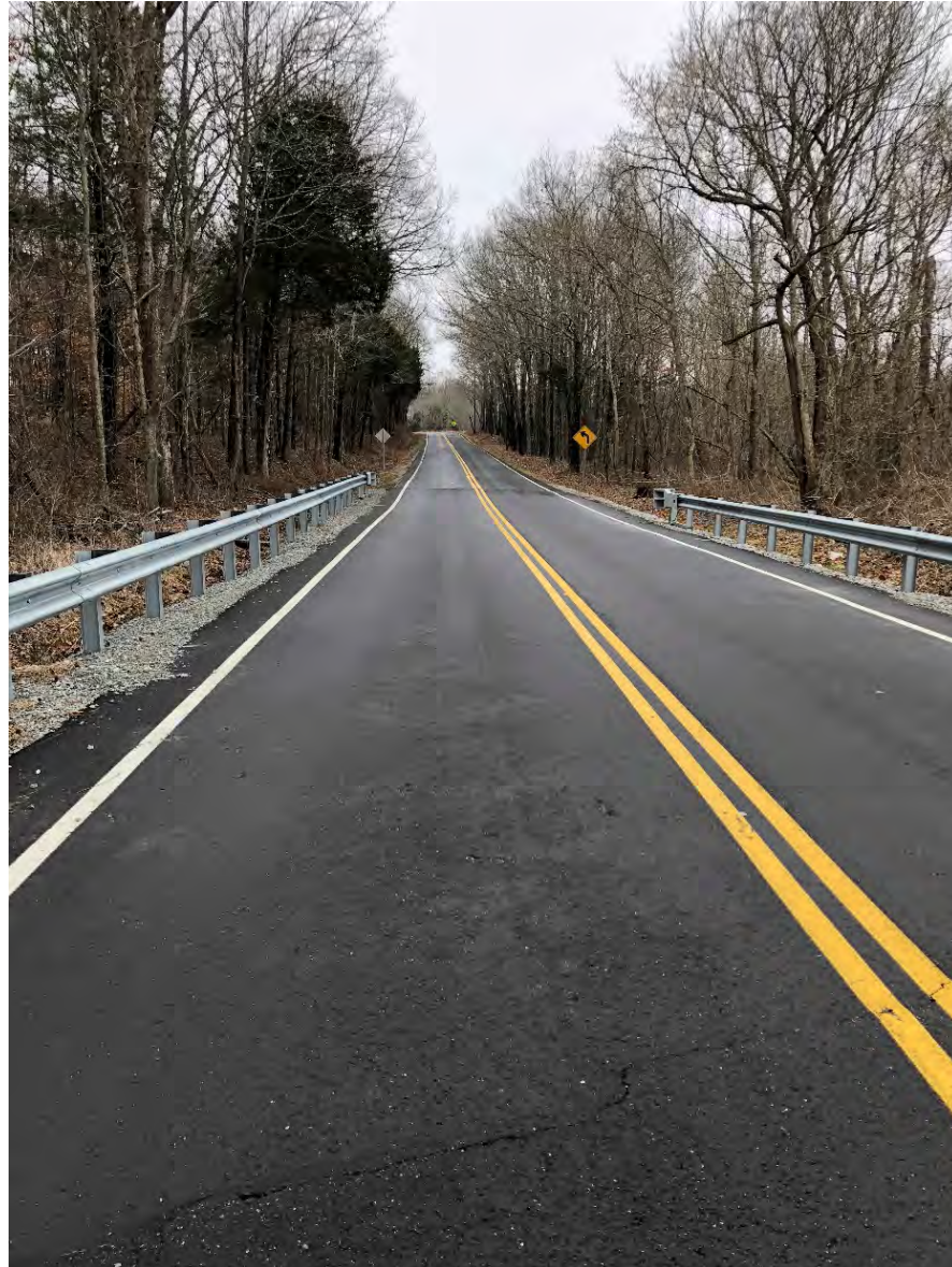
Looking East from Bridge
